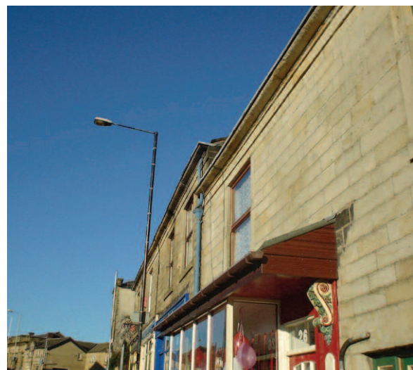
Integral troughing on Church Street shops
