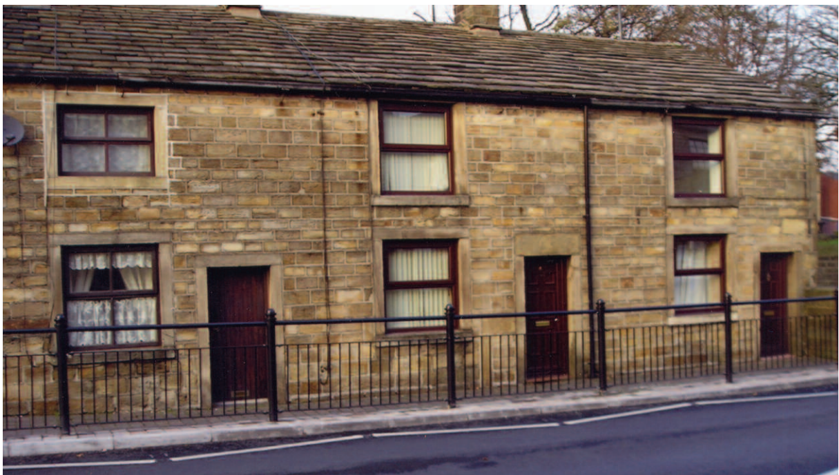
Falcon Cottages illustrating typical door frames
