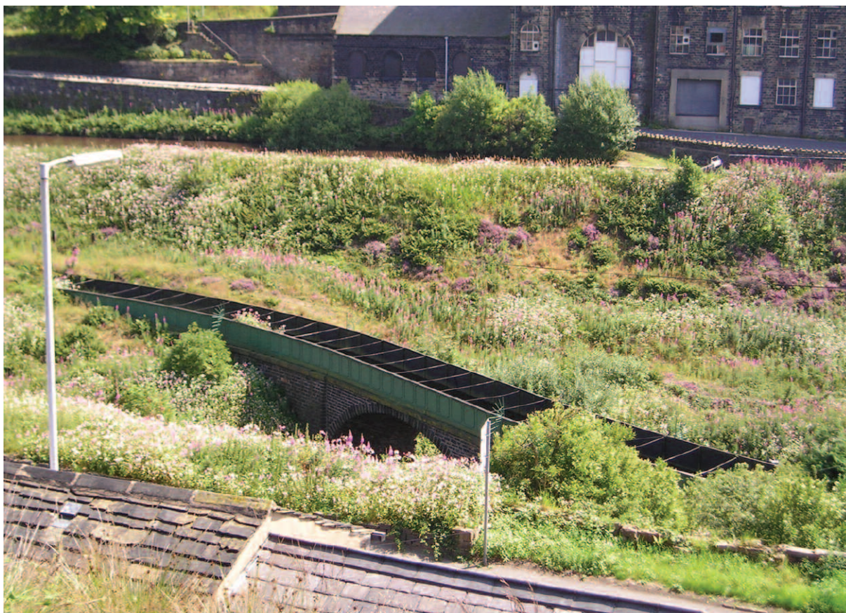
Summit - cast-iron aqueduct carrying the River Roch over the railway
