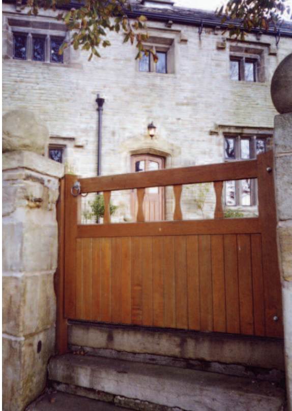
Shore Hall illustrating drip mouldings
