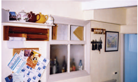
Calder Cottage showing former external window, now inside
