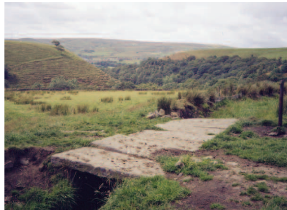
Stone slab bridge
