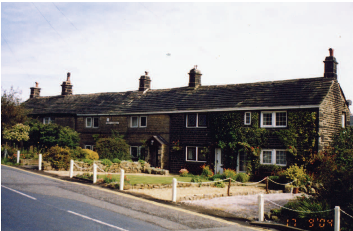
Cottages at Lower Calderbrook
