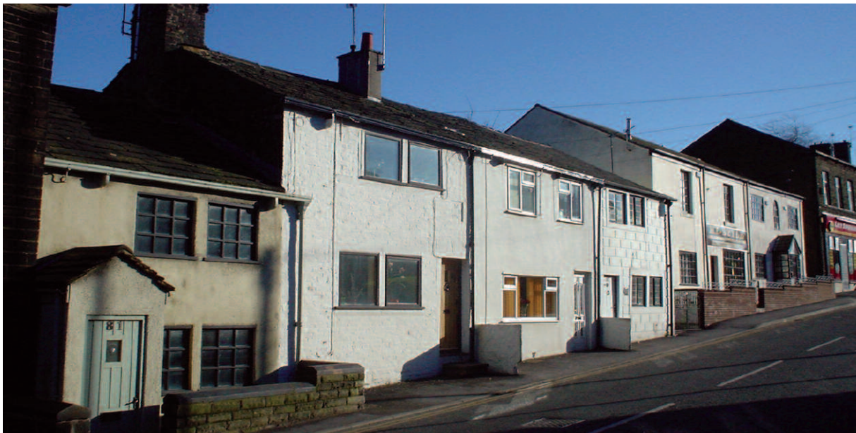
Cottages at Smithy Bridge
