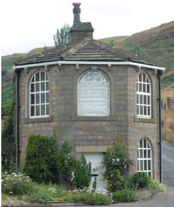
Steanor Bottom Toll House
