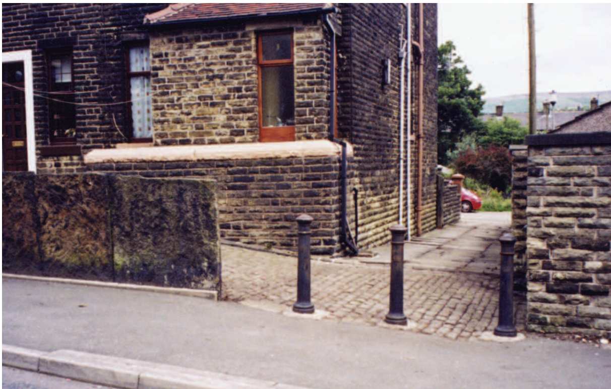
Original flag walling, setts and cast-iron bollards on Lodge Street
