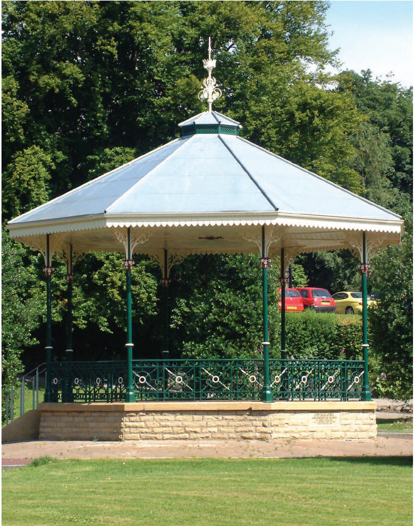
The bandstand in Hare Hill Park, refurbished 2004
