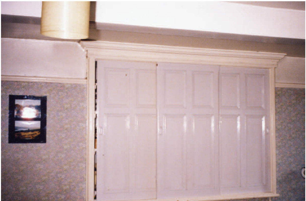
Calder Cottage showing former external window, now inside
