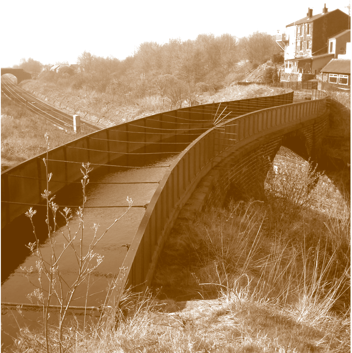
(Above) Stephenson's aquaduct carrying the river Roche over the railway line
